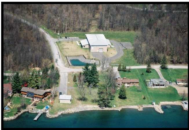
Long Sault Intake, South Stormont
